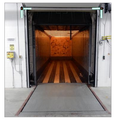
Mounted on the interior wall above the top two corners of the dock door, the lights extend out along the edges of the dock door opening to provide a visible indication when it's safe to enter the trailer.
