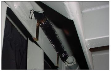
When the brush is pressed into place it is supported by the metal clips. The brush expands sealing the void between the rear header and the hinge where air and rodents could enter.
