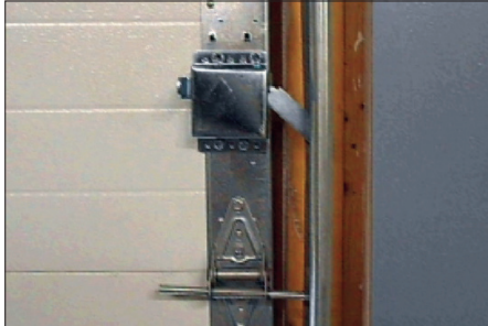
Traditional lock under pressure fails
